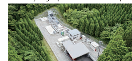
Green Hydrogen production verification plant
