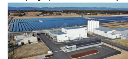
Hydrogen production research facility
