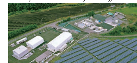
Yonekurayama Electric Power Storage Technology Research Site
